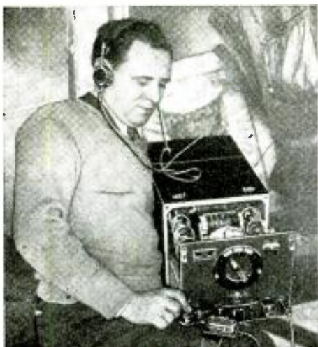
Appearance of the new Aircraft transmitter. No. 302
